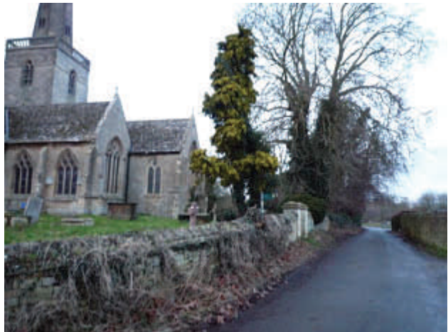
Limestone boundary wall at the church
