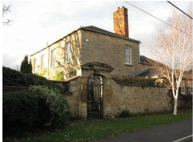
Manor Farm, 17 Church Street
