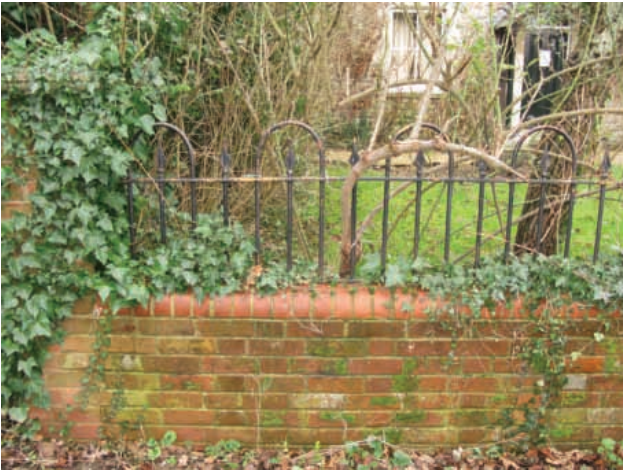
Wall and railings at 28 School Road
