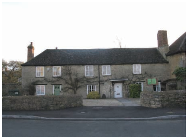
The former workhouse, 14 School Road
