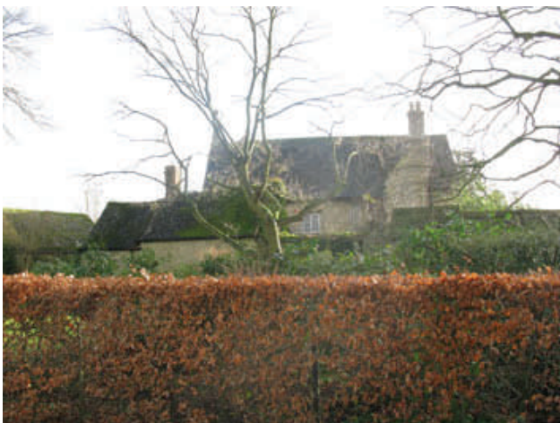
Buildings are hidden from the main carriageway
